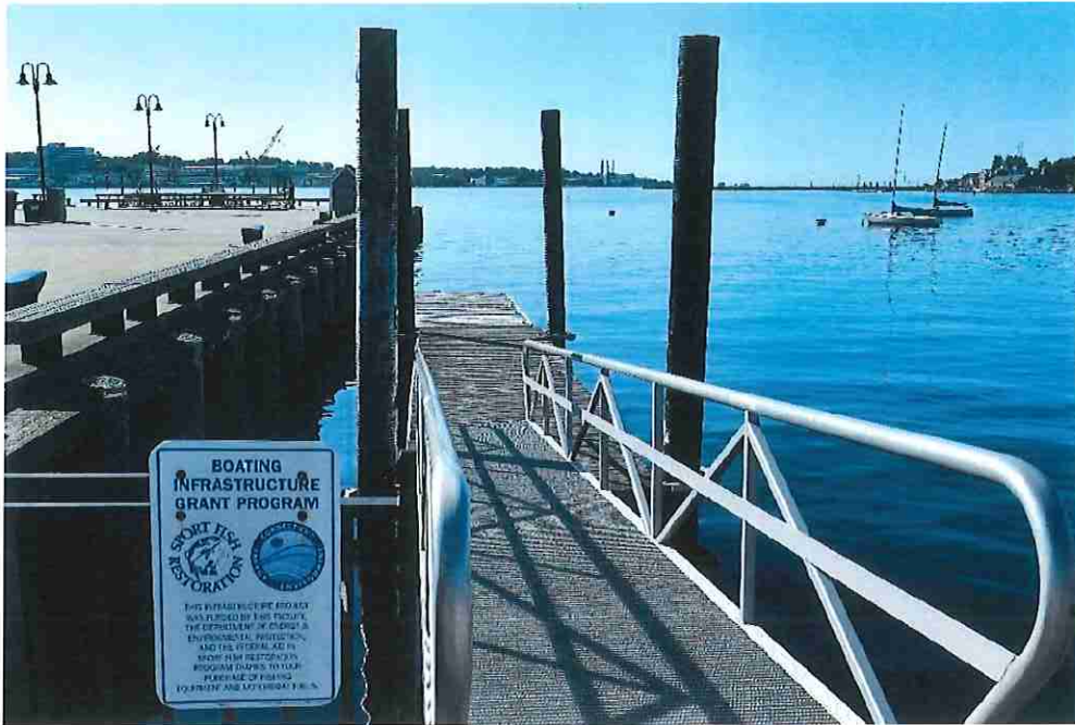
Photo 4: Custom House Pier Concrete Piling
