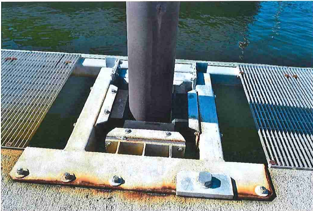
Photo 9: Floating Dock Pile Guide
