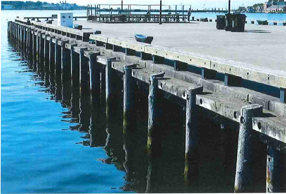
Photo 1: Custom House Pier North Bulkhead
