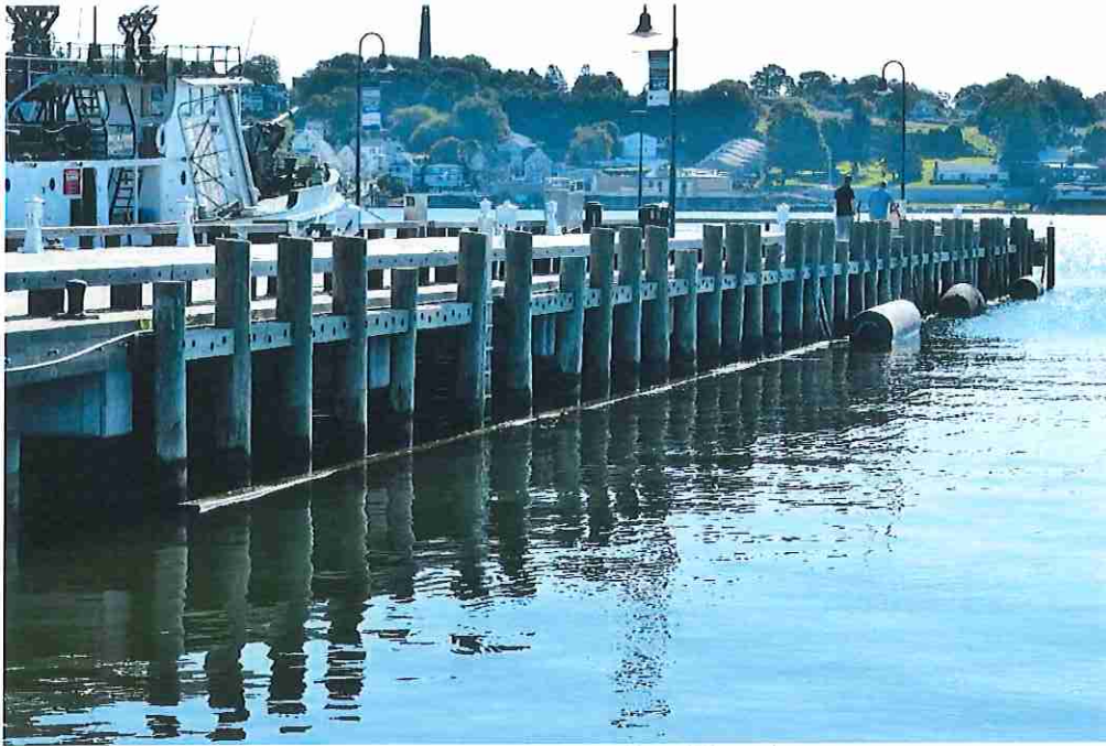
Photo 6: City Pier South Bulkhead
