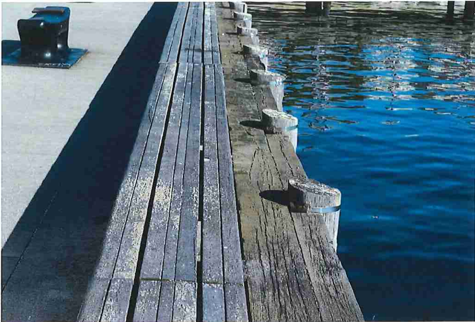
Photo 3: Custom House Pier Bulkhead
