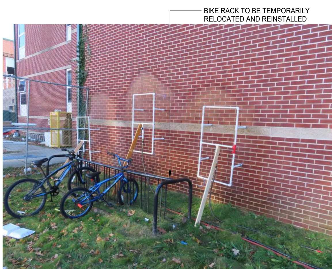
4 PHOTO OF WORK AREA NEAR SOUTHEAST END SCALE: NONE
