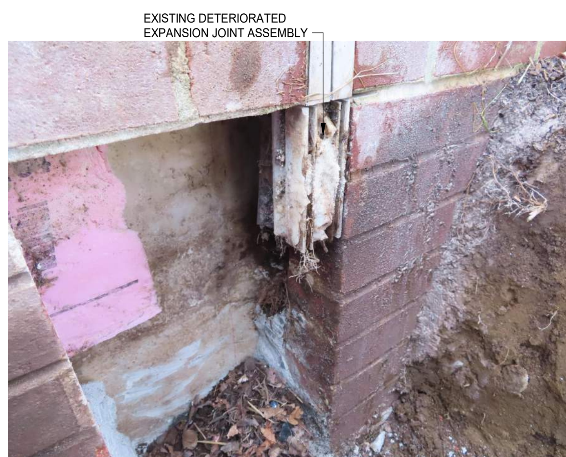
9 PHOTO OF TEST CUT AT EXPANSION JOINT SCALE: NONE
