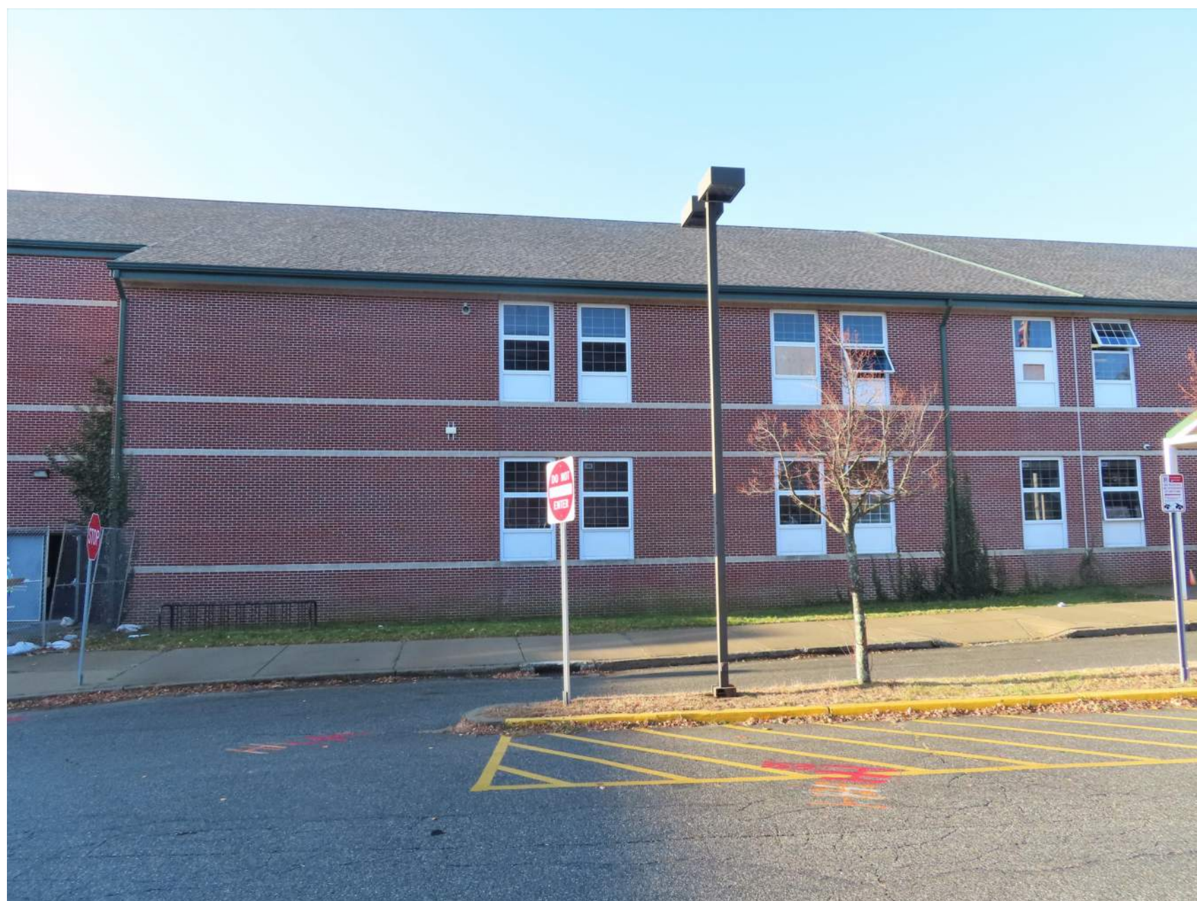
1 OVERALL PHOTO OF WORK AREA AT NORTHEAST ELEVATION SCALE: NONE
