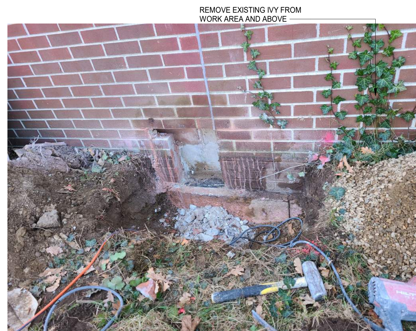
6 PHOTO OF EXCAVATION AND TEST CUT AT CONTROL JOINT SCALE: NONE
