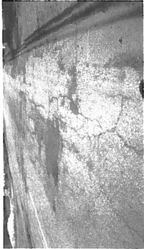
Cracking/Settling/Subbase Failure #3
