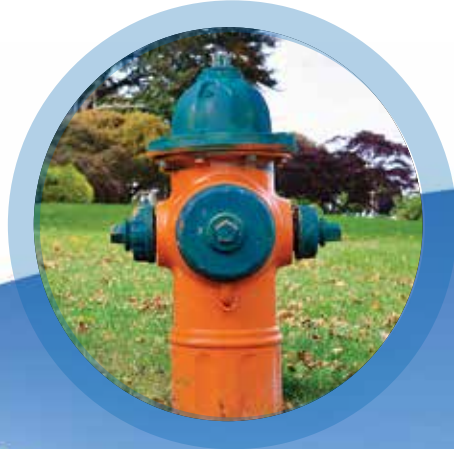
Maintenance of 2,000 hydrants
